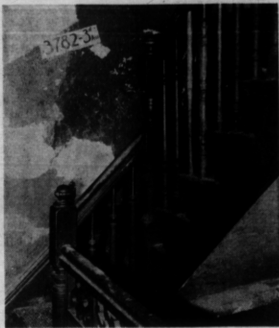
CRACKED WALLS IN A HARLEM TENEMENT
